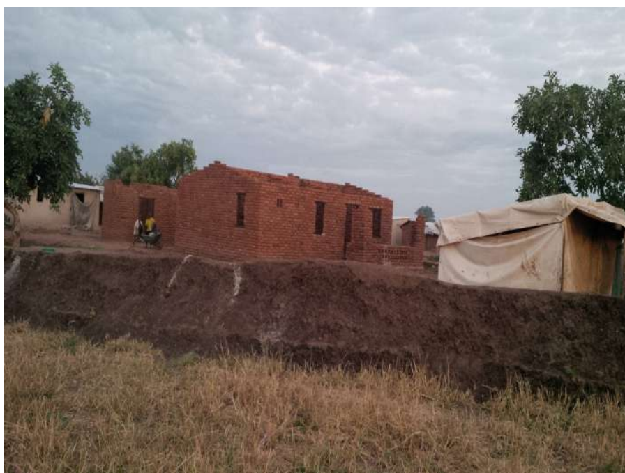
Figure 2 An earth dyke constructed by communities at a new resettlement site in Chikwawa to prevent flooding
