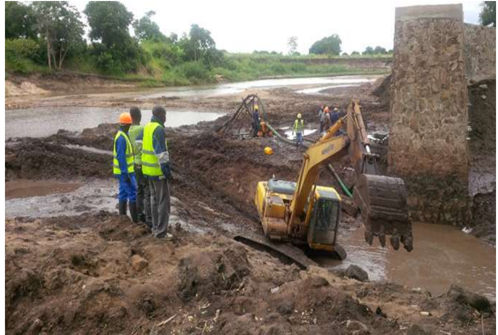
Figure 1: The most visible aspects of recovery; reconstruction of a washed away bridge in Phalombe District
