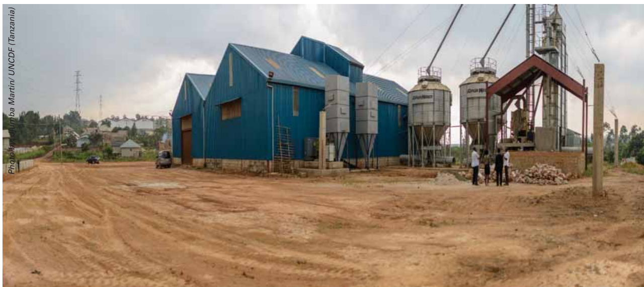
The NUCAFE factory in Namanve Industrial Park in Mukono District, Uganda.
