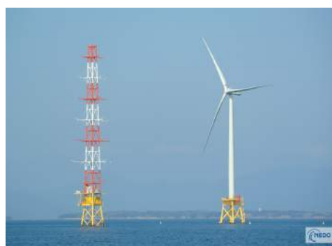
Wind power generation
