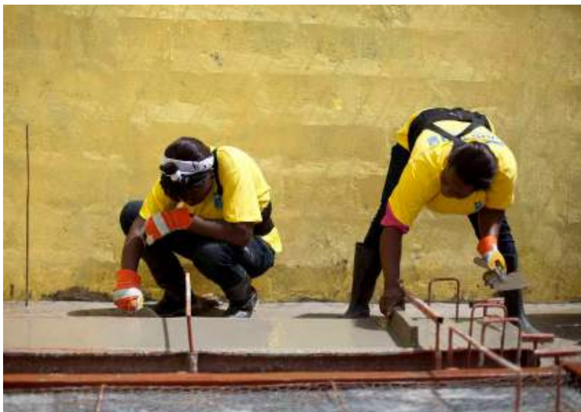
UNDP Andres Martinez Casares Women working in the CARMEN House self-repair Project
