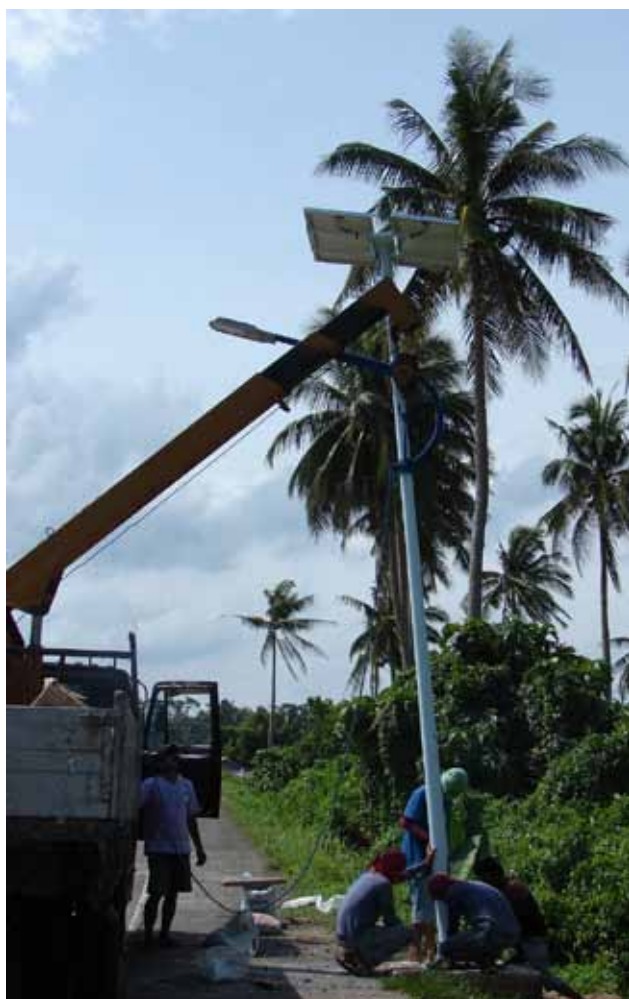
Installation of a solar-powered street light along Diversion Road in Sorsogon City, Philippines.
