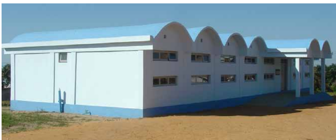
Cyclone-proof kindergarten in Vilankulo, Mozambique. © UN-Habitat/Arianna Francioni
