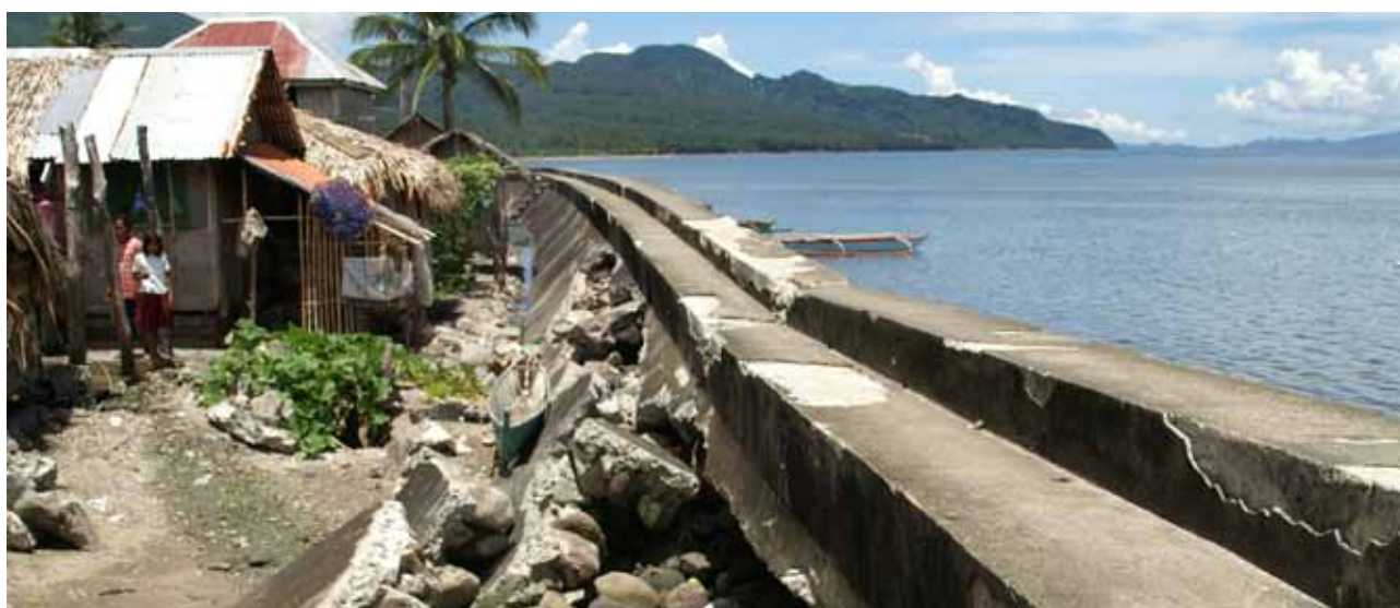
Seawall in Sorsogon City, Philippines © UN-Habitat/Bernhard Barth
